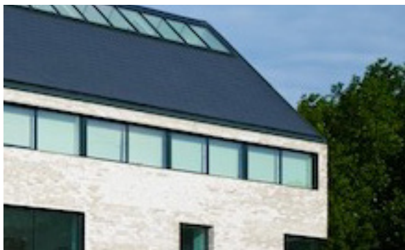
Fibre cement slate roof
