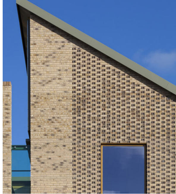
Feature panels of textured brickwork
