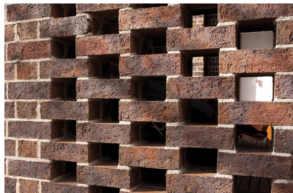
Hit and miss brickwork to circulation areas
