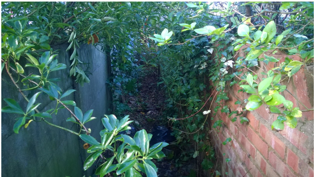
Narrow path along rear of 91, 93 and 95 Crewys Road accessed from gap between 91 and 87 Crewys Road.
