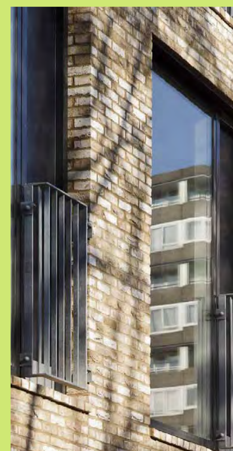
Example of balcony and fenestration treatment
