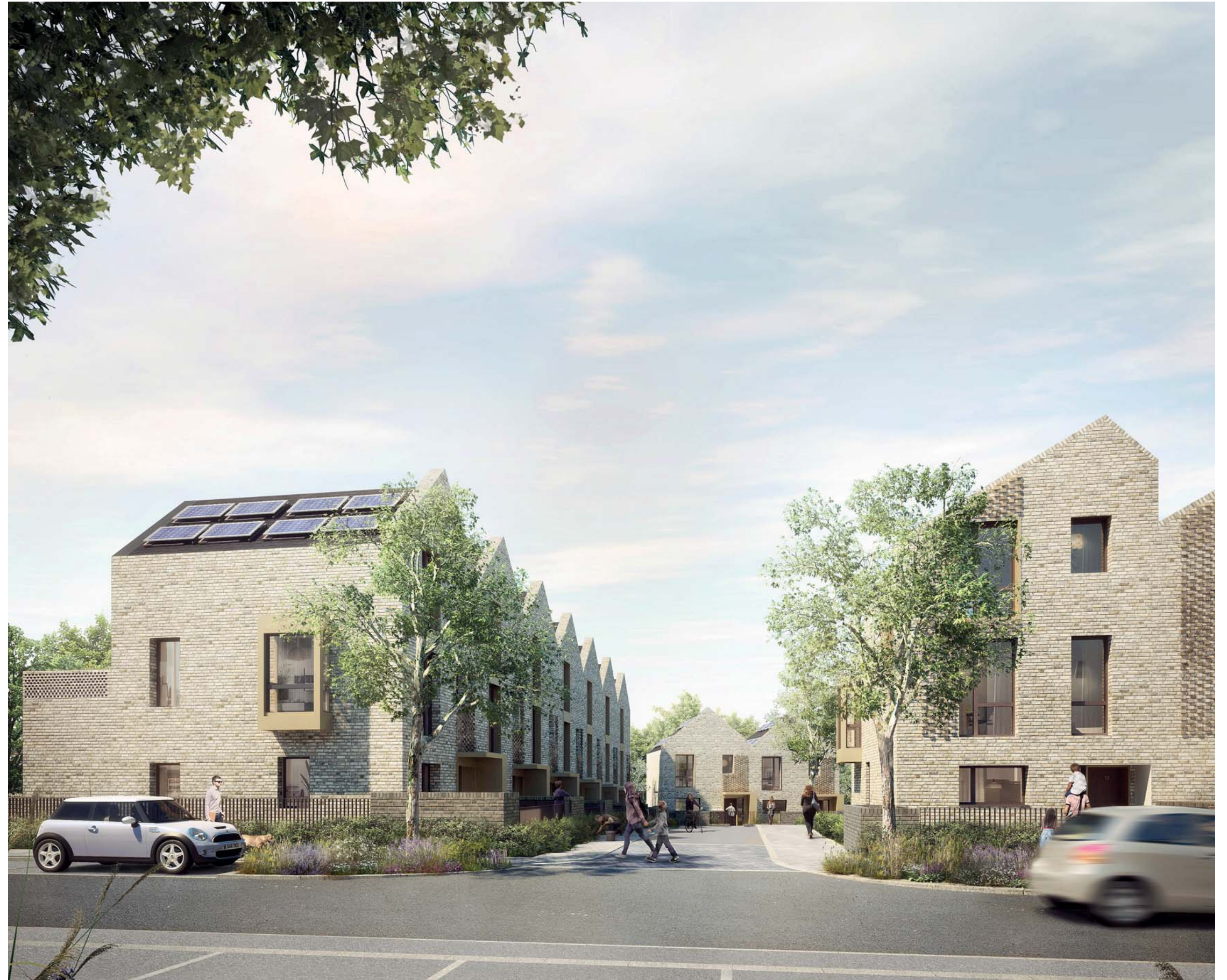
02 View looking west into 'The Close' from Granville Road
